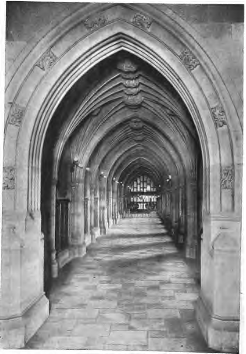
7. THE EAST CLOISTER
